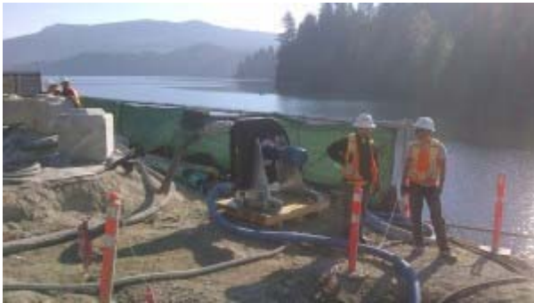
An 80mm pump on Drilling mud
